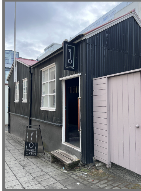
Fig. 2: Fischersund, the shop. Located in a 19th century building that has been refurbished but retains old world charm.
